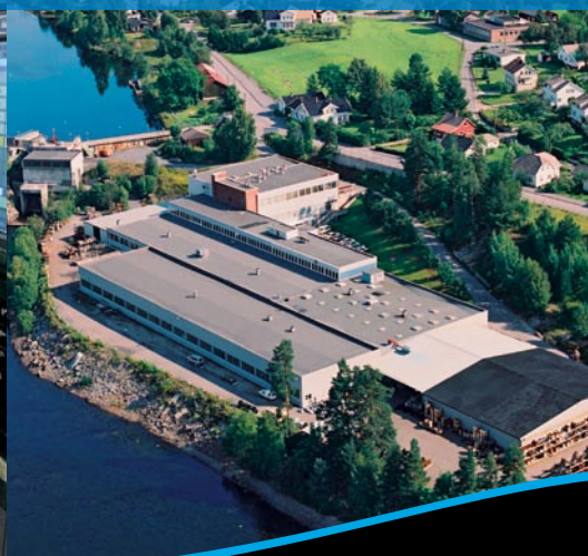
Production plant in Kongsberg.
